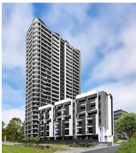
First Meriton tower, the smallest of the four planned for the site
